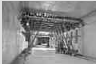
Tunnel Formwork
