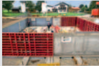
Wall Formwork
