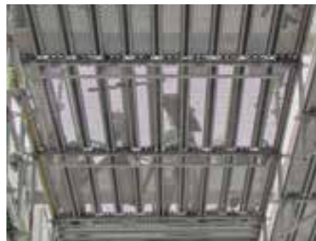
Platform completely covered with PERI UP system decking.
