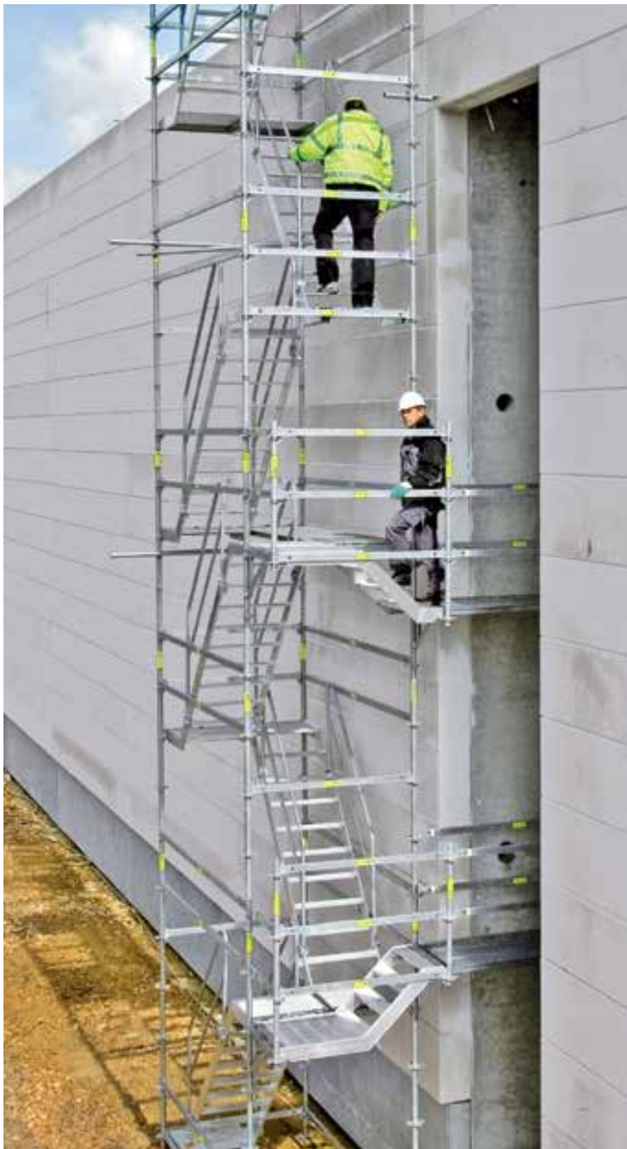
Height adjustments on building openings are installed independent of the floor height.
