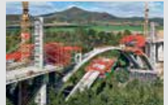
Bridge Formwork
