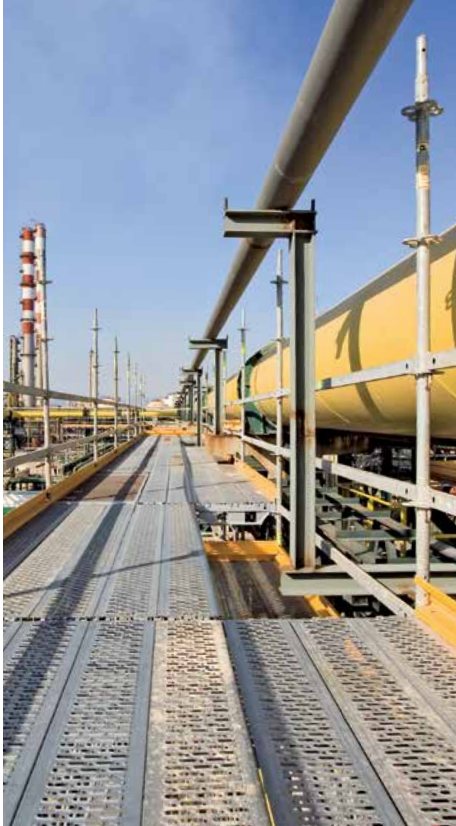
Lightweight ledger used as a guardrail. For platforms, reinforced or standard ledgers are used depending on the load requirements.
