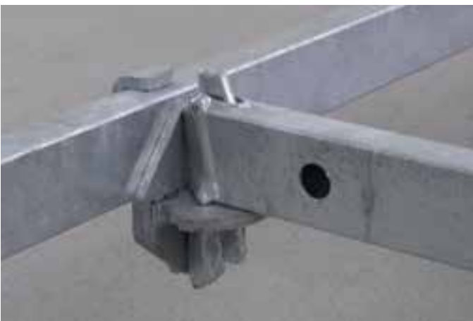
Ledger-to-ledger connecton.
