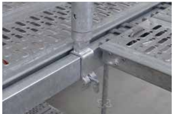
Standard-to-ledger connection.
