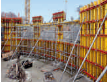
Use with VARIO GT 24 Girder Wall Formwork The Arctic Ring, Copenhagen Zoo, Denmark.
