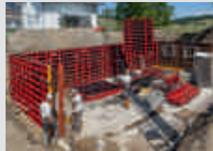
Wall Formwork
