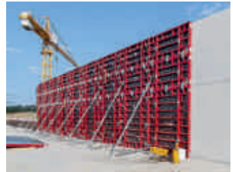
... and installation at the required position.
