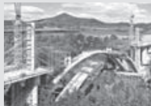
Bridge Formwork
