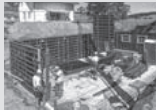
Wall Formwork
