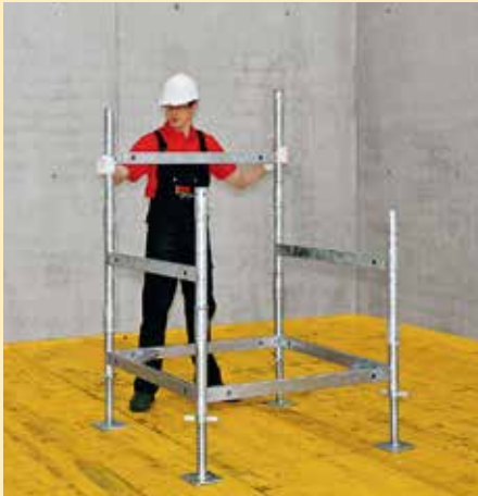
Install required number of stacking frames.
